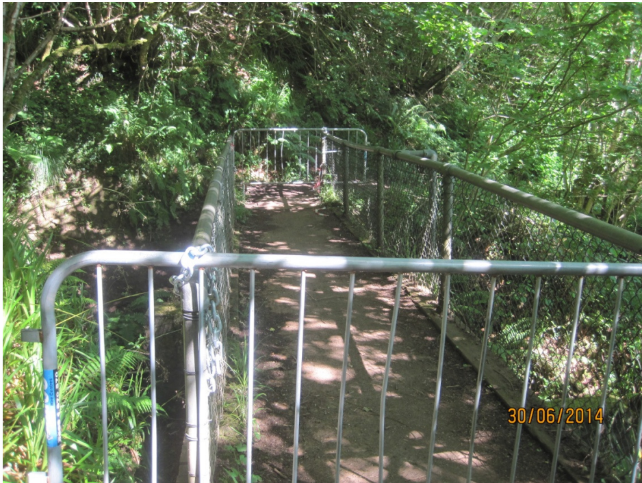
Figure 5 Overview of Bridge
