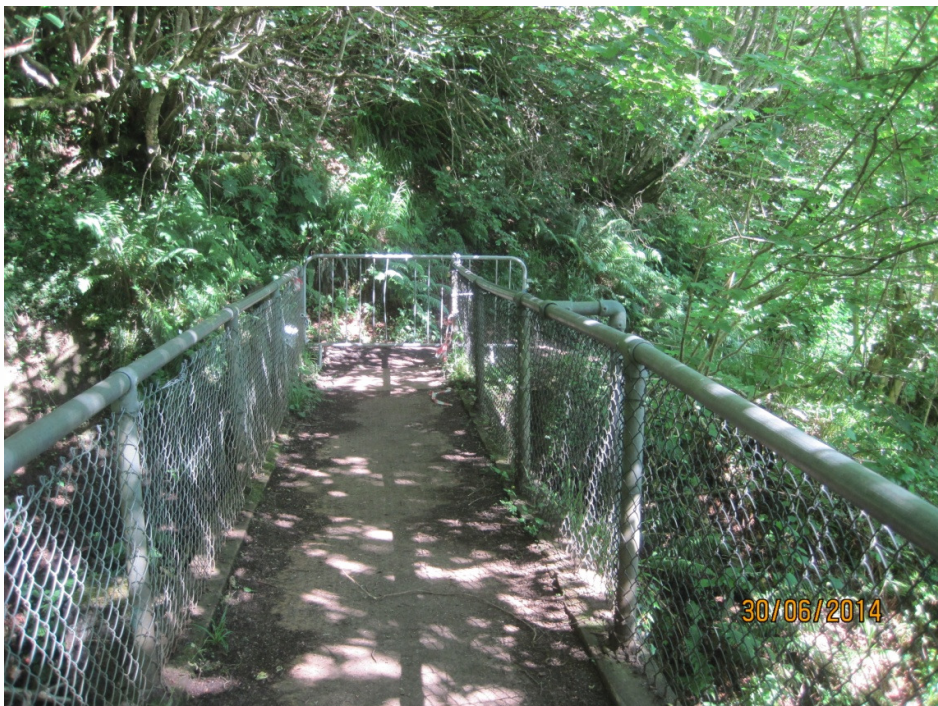
Figure 6 overview of Bridge
