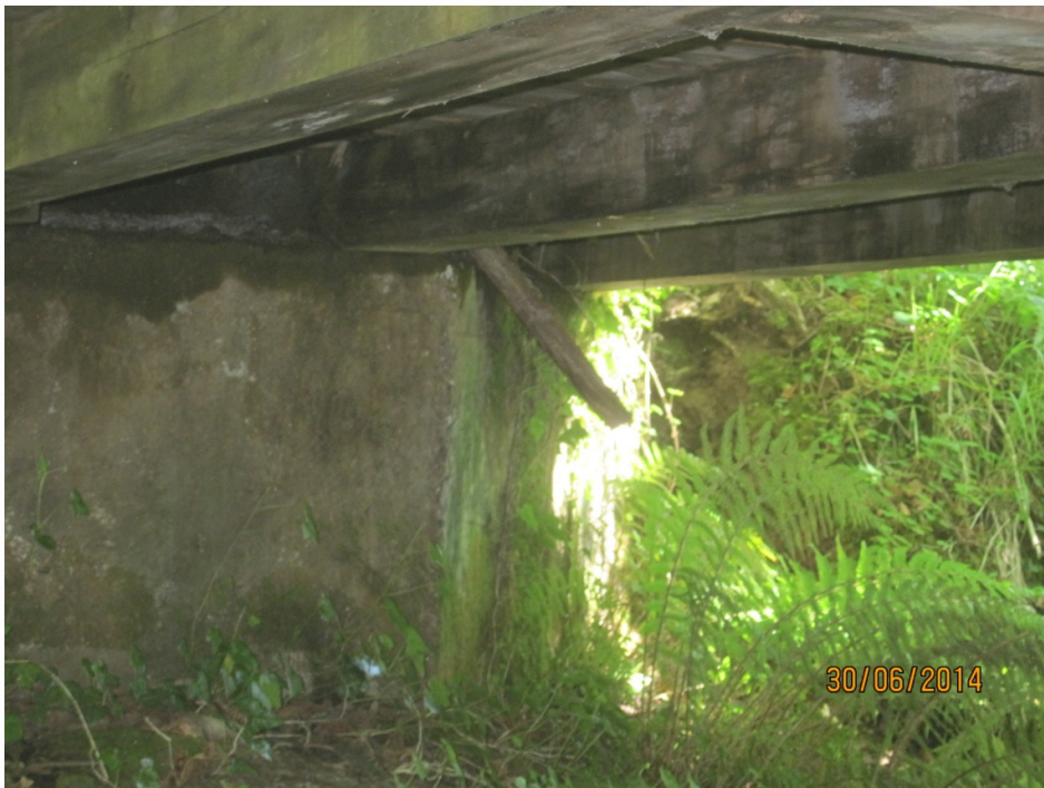
Figure 4 View of underside of bridge
